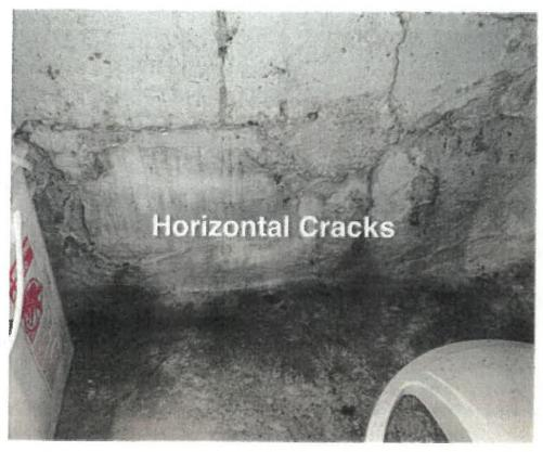
Horizontal cracks are the most serious. It may be that water-saturated soil froze and expanded, pushing in and breaking the foundation. Or, you may have soil that expands when damp, and shrinks when dry. The bad news: You probably need to repair part, if not all, or your foundation.
